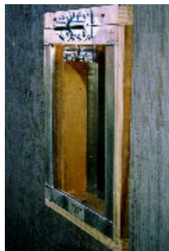
This is how an installed door looks.
